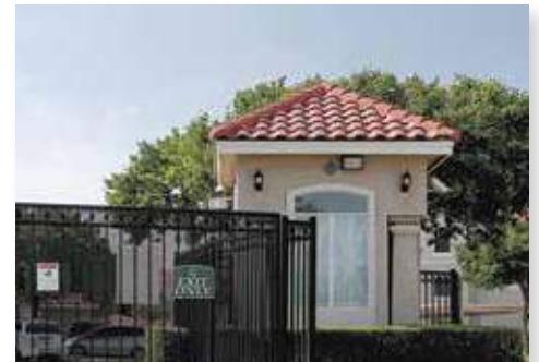
Backup Access at Gate House
